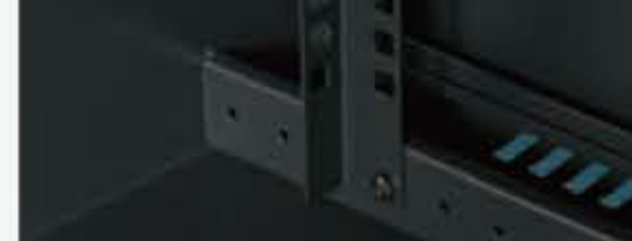
High precision installing mounting profile
